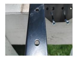
7. Affix mailbox to mounting plate using bolts, washers, and nuts provided. This is how it would look from the bottom of the box before being mounted, with the washers and nuts on the bottom.
