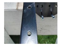
7. Affix mailbox to mounting plate using bolts, washers, and nuts provided. This is how it would look from the bottom of the box before being mounted, with the washers and nuts on the bottom.
