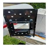
4. Place plate on post arm and mark the two holes at the bottom of each post adapter on the post arms with a pencil. (see pictures below)
